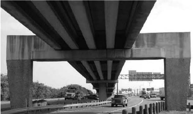
FIGURE 5.13 Bent cap.
